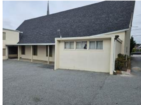
South side of the building was power washed and scrubbed clean July 2024
